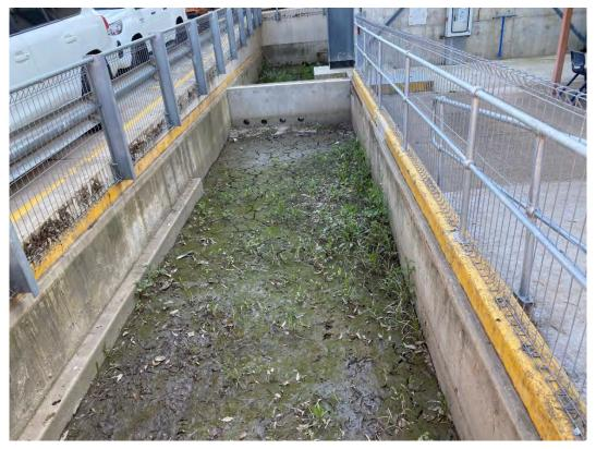
Plate 18 - Stormwater sandfilter system
