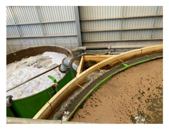
Plate 8 – Scum tank separating clean water before discharge to sewer through TWA
